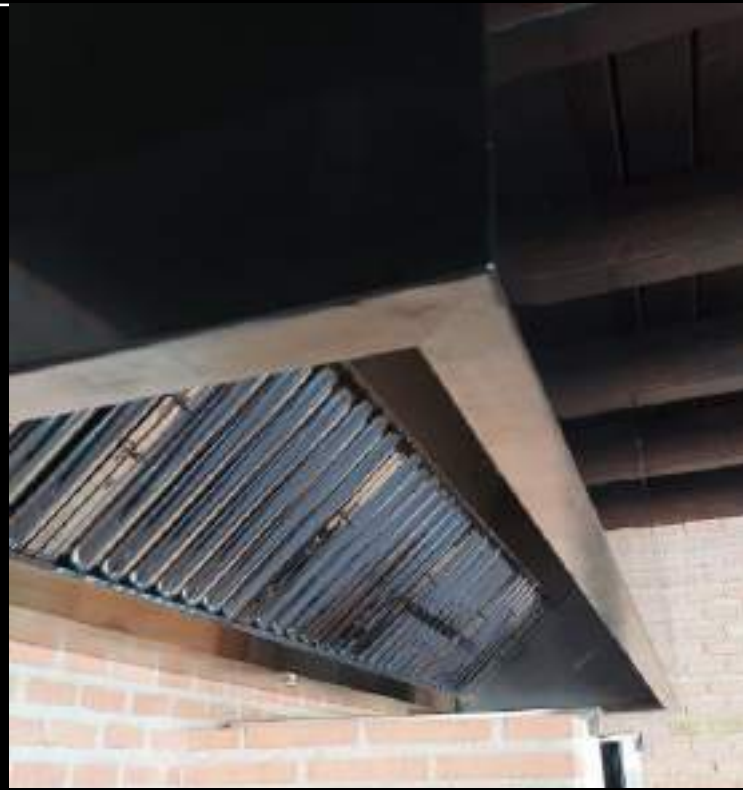
HOOD WITH FILTERS UP TO 1300MM
