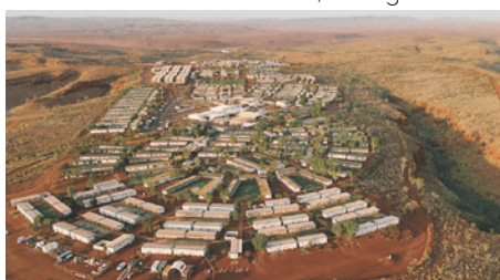
Operational and design experience remote accommodation and catering.
